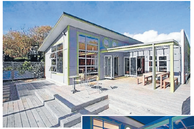
Otaki: Clients wanted a beach bach in their new build with a strong sense of connection to the rear garden; silver corrugated steel and painted battened cement sheet connects with materials used in original Raumati bachs.
